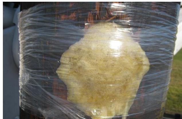
Woodpecker damage repaired with UPR™ Pole Repair
