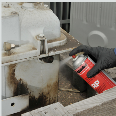
Removing transformer oil residue
