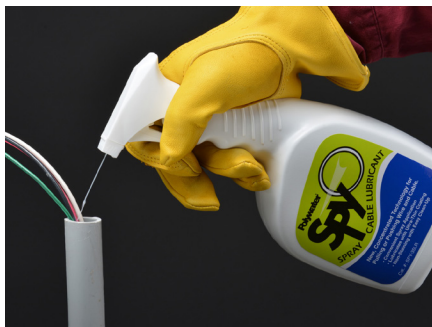
Applying SPY lube to THHN
