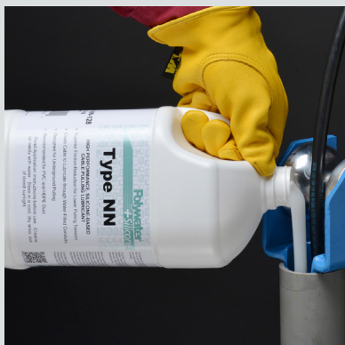
Pouring lube into a conduit stub-up
