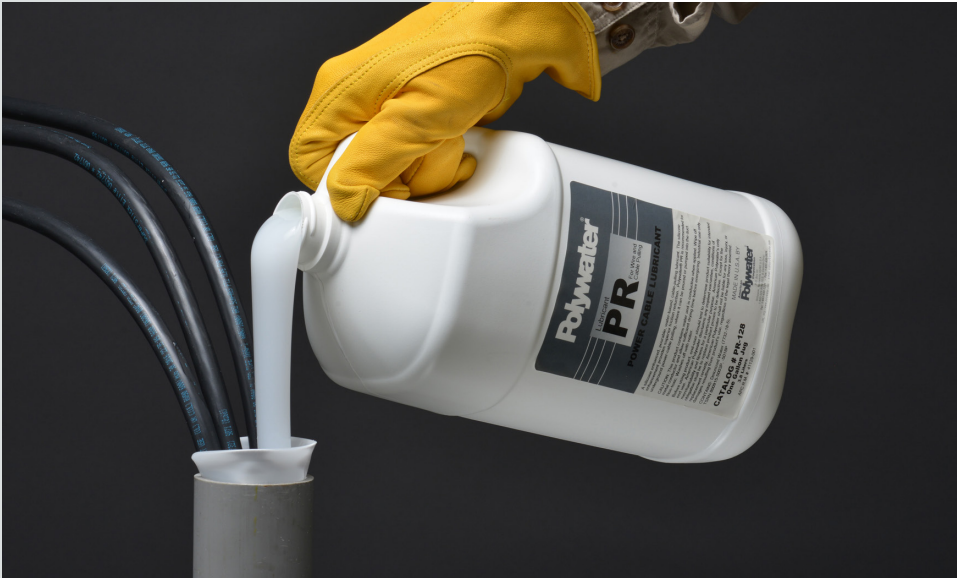
Pouring PR into a conduit stub-up
