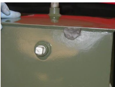
Clean area with cleaning wipe before applying Polywater ® Putty Stick
