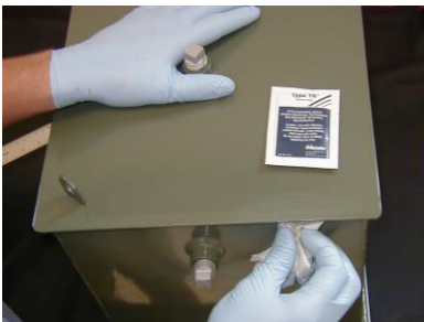
Clean area with cleaning wipe before applying Polywater ® Putty Stick
