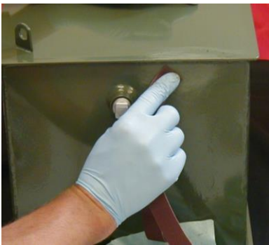
Sand or brush repair area
