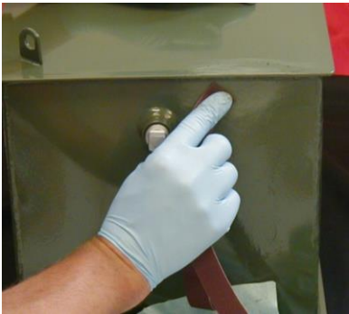
Sand or brush repair area
