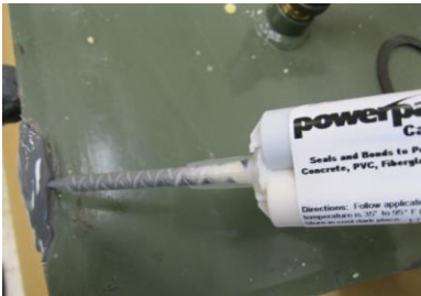
Apply PowerPatch® Sealant over Polywater® Putty Stick patch or leak area
