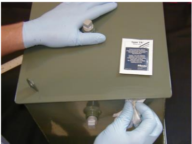
Clean area with cleaning wipe before applying Polywater ® Putty Stick
