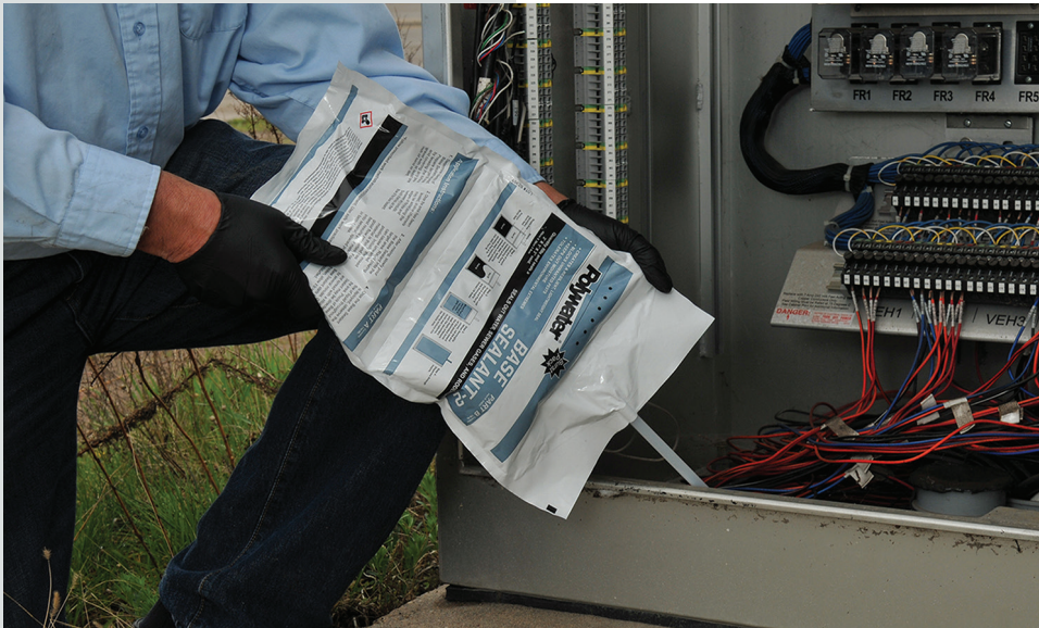
Polywater PedFloor burst pack installation
