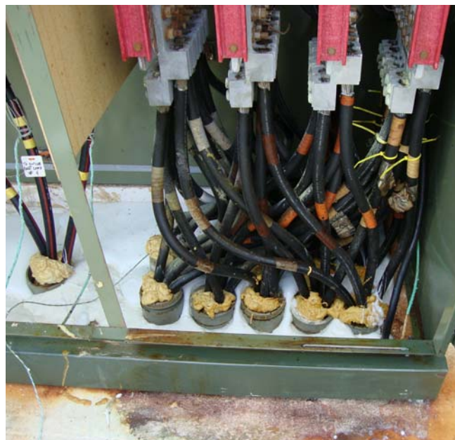
InstaGrout™ Sealant is used to fill a transformer cabinet base in place of concrete.
