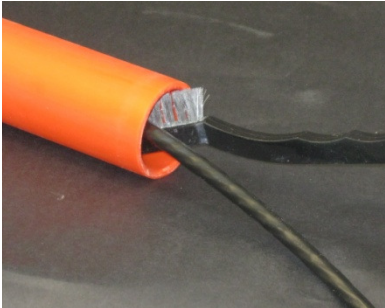
Clean duct with wire brush.
