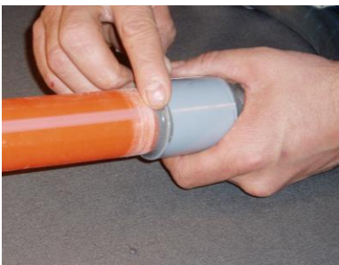
Smooth Excess Material
