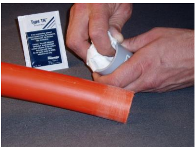
Clean Coupling and Conduit with Cleaning Wipe
