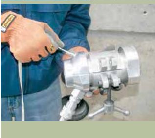
Install pulling tape into winch blower through \frac{1}{16} " tape adapter.
