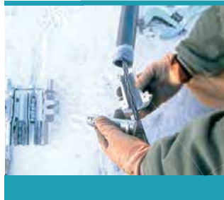
Install the winch line in the conduit and thread adapter into conduit.
