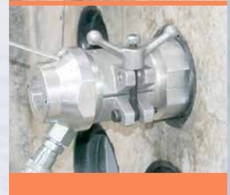
Complete the assembly and blow in tape.
