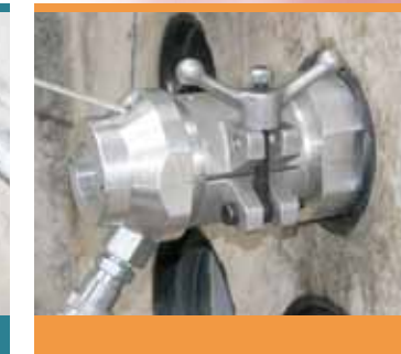
Complete the assembly and blow in tape.
