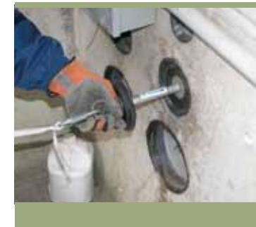
Attach tape to carrier and insert carrier into pipe.
