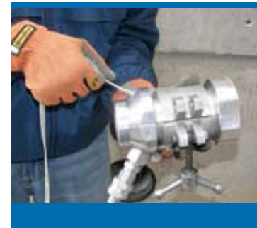
Install pulling tape into winch blower through 7/16" tape adapter.
