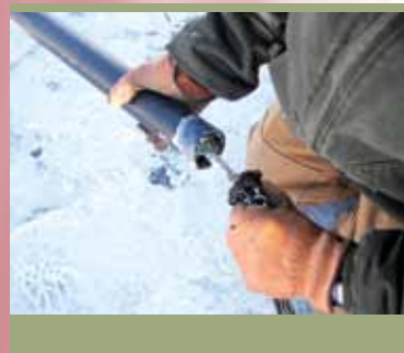
Attach winch line to carrier and insert carrier into pipe.
