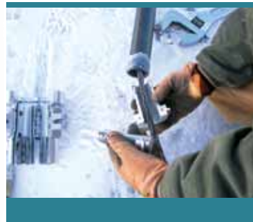
Install the winch line in the conduit and thread adapter into conduit.
