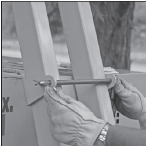
Figure 2. Remove Traveling Pin
