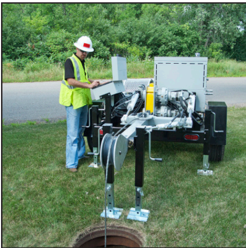
Figure 6. Monitor Pulling Tension and Distance
