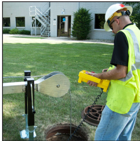
Figure 7. Use Joystick to Increase the Pullback Speed
