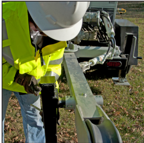
Figure 2. Lower Arm and Install Jacks
